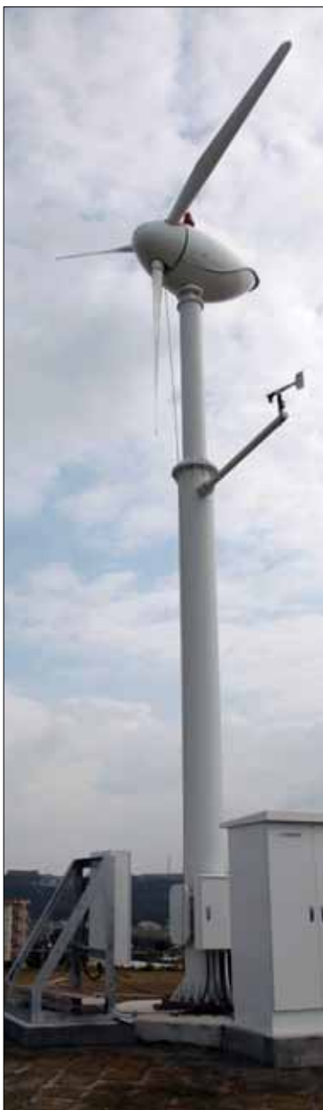
Japanese contractors recently constructed one of the Department of Defense's first wind turbines in Japan adjacent to Building 1 on Camp Foster. The turbine is expected to be fully operational in mid-April and will generate clean power and help reduce MCB Camp Butler's carbon footprint and utility costs, according to Tomoko Matsuzaki, an energy engineer with facilities engineers. Photo by Lance Cpl. Brandon C. Suhr
