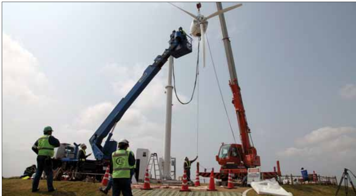
A wind turbine is installed March 19 adjacent to Building 1 on Camp Foster. The turbine is capable of generating 10 kilowatt-hours each hour at its peak, which, as an example, would power the fluorescent lights on one floor of Building 1, according to Capt. Steven M. Bancroft, energy and utilities officer in charge with facilities engineers, G-F, Facilities, Marine Corps Base Camp Smedley D. Butler, Marine Corps Installations Pacific. Photo by Lance Cpl. Brandon C. Suhr
