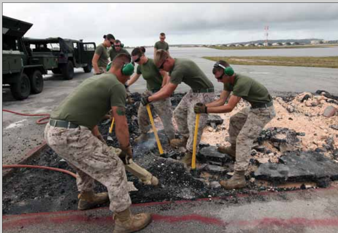
Marines repair pavement March 21 at Andersen Air Force Base on Guam during Exercise Guahan Shield. Marines repaired sections of the pavement for use in future training. The Marines are assigned to Combat Logistics Detachment 39, 3rd Marine Logistics Group, III Marine Expeditionary Force. Photo by Lance Cpl. Jeraco Jenkins
