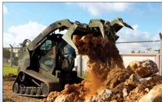
Lance Cpl. James S. Sipper uses a multiterrain loader to pile rocks and debris July 8 during the removal of a 60-meter-long wall near U.S. Army Garrison Torii Station's main gate. Sipper is a heavy-equipment operator with 9th Engineer Support Battalion, 3rd Marine Logistics Group, III Marine Expeditionary Force.
